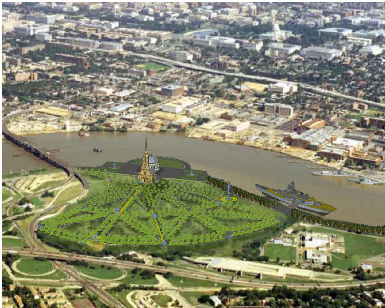
Picture 1. A bird’s eye view from a southeast vantage point
